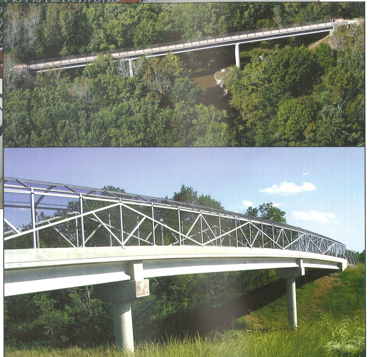
JUDY BALES Cedar View Trail Bridge. Self-weathering steel. Design for steel elements retrofitted to existing bridge, laser-cut art elements installed by community volunteers. Each element 5.5' high, bridge span 385'. BELOW: JUDY BALES Cedar View Trail Bridge. Aerial view.
